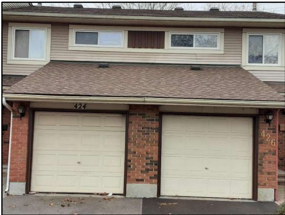
View of architectural shingles.
