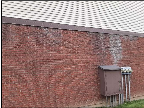
View of efflorescence on brick veneer.
