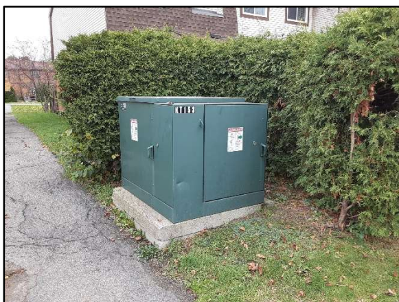
Typical pad-mounted transformer.
