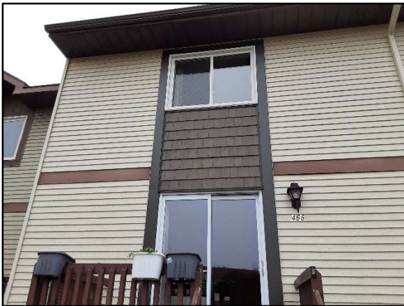
View of shakes siding.
