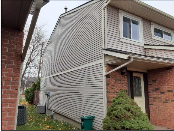
View of aluminium siding.
