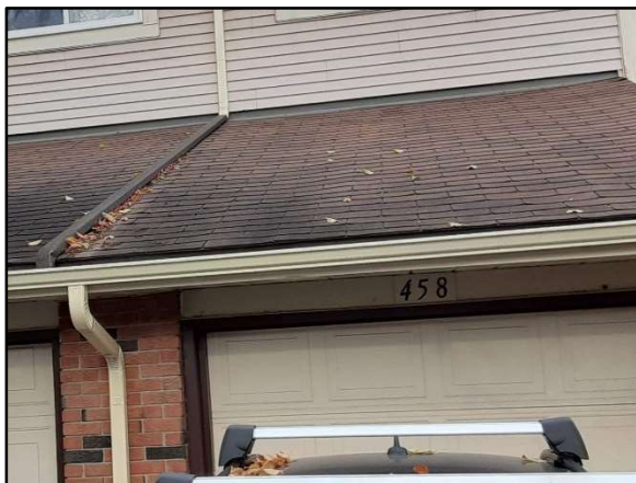
View of 3-tab shingles.
