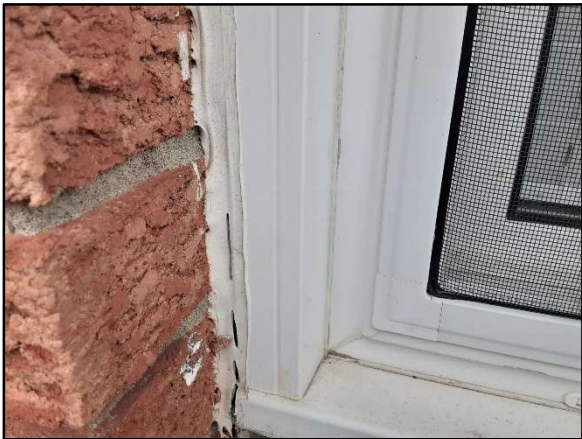
View of typical window perimeter sealant.
