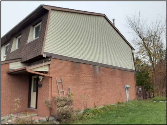
View of efflorescence on brick veneer.
