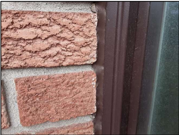
View of typical door perimeter sealant.
