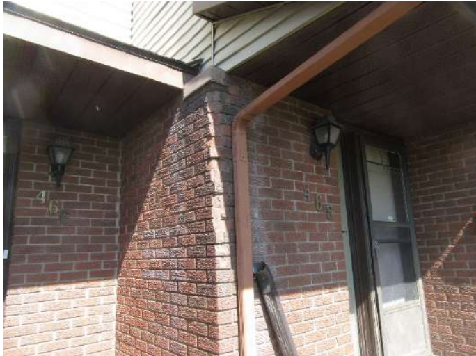
Photo B.7 – Showing spalled bricks.
