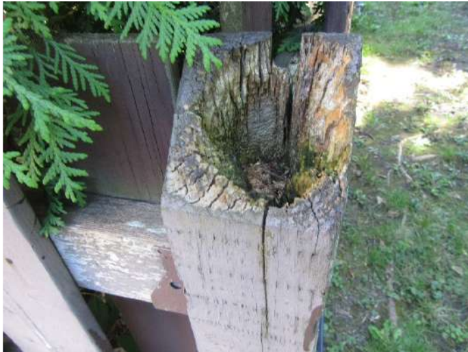
Photo B.5 – Deteriorated post at a privacy fence.
