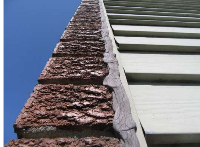
Photo B.8 – Showing deteriorated caulking at cladding junction.
