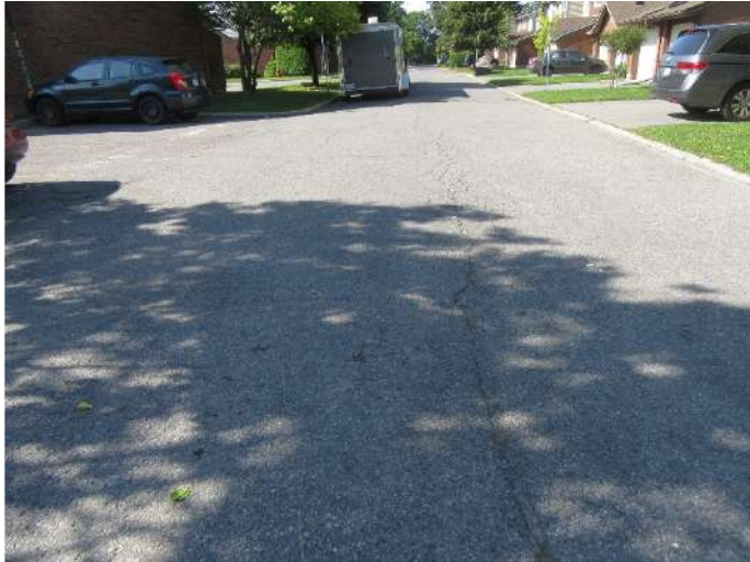
Photo B.3 – Showing longitudinal cracking through roadway asphalt pavement.
