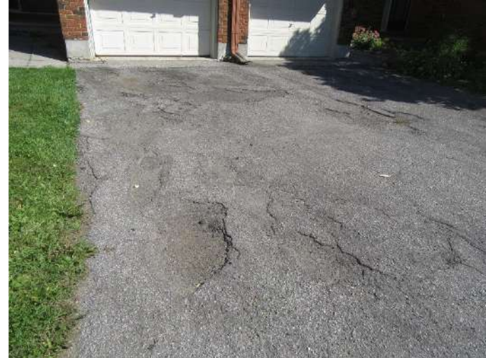
Photo B.4 – Showing depressions and deterioration of the asphalt pavement at a driveway.
